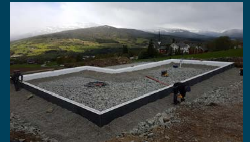
Ringmur for foundations
